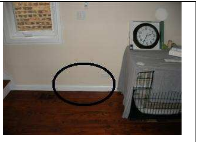
Picture 16. Exterior wall
