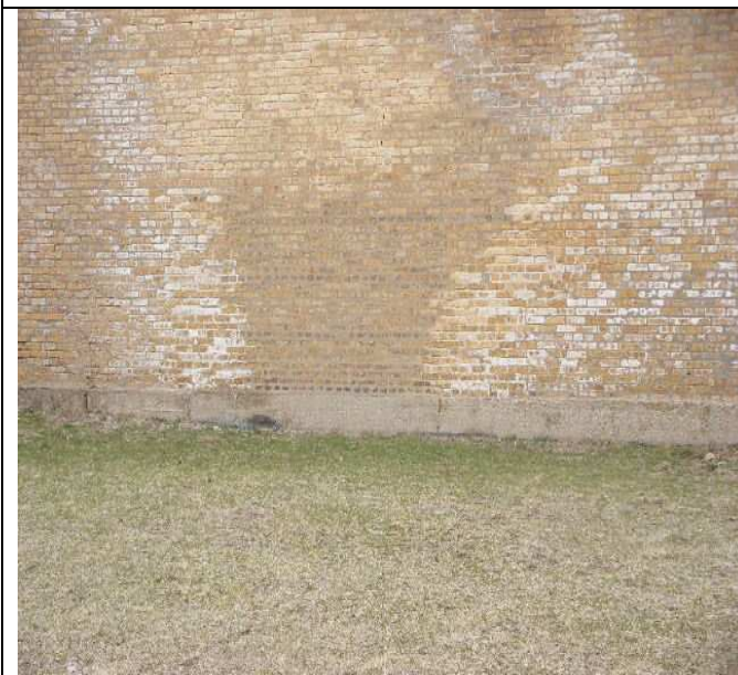
Picture 5. Wicking water efflorescence
