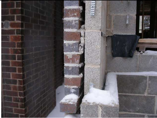
Picture 9. Mortar bridging the intra-wall gap
