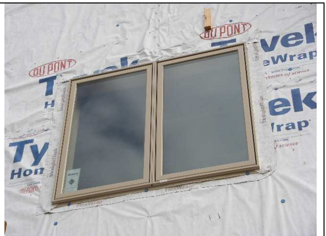
Picture 12. Proper window taping detail
