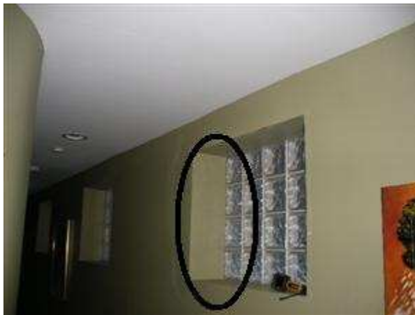
3.2 Picture 3 Basement, North wall
